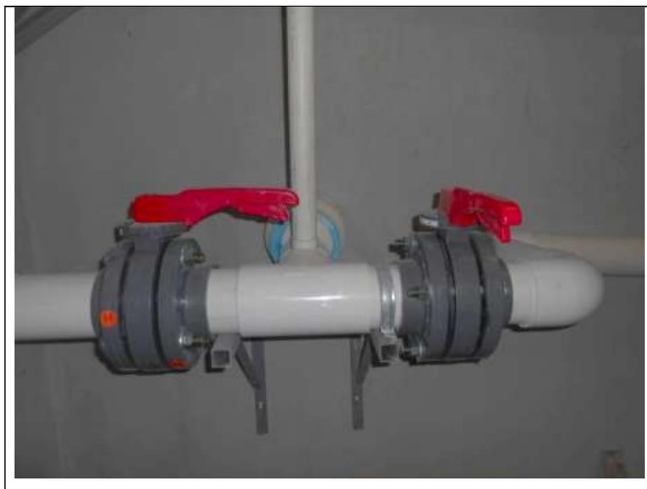
Figura 40 Bypass instalado
